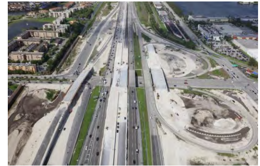
SR 836 WESTBOUND BRIDGES AT 87 TH AVENUE
