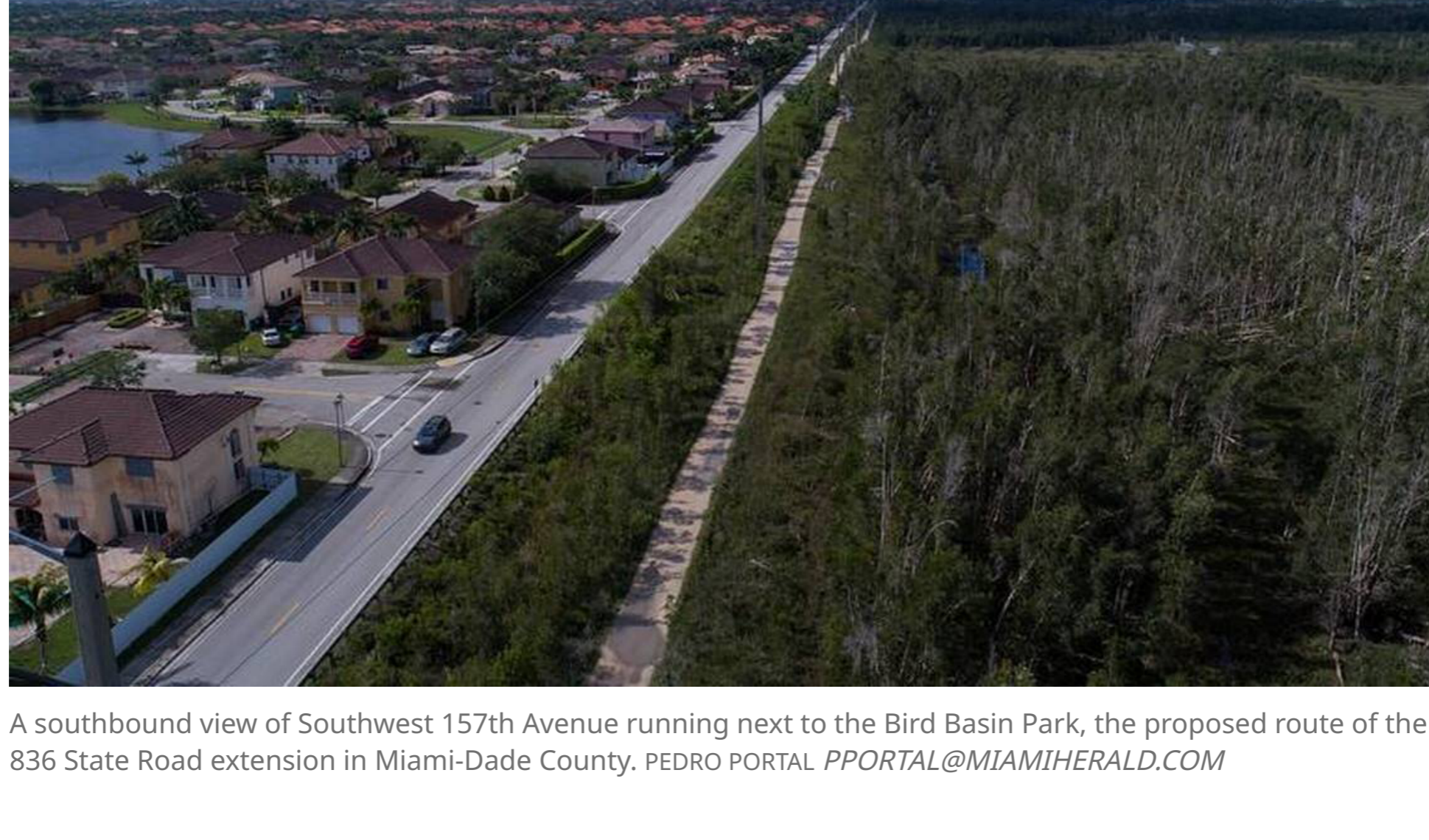
A southbound view of Southwest 157th Avenue running next to the Bird Basin Park, the proposed route of the 836 State Road extension in Miami-Dade County. PEDRO PORTAL PPORTAL@MIAMIHERALD.COM
