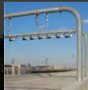
Distance-based charge for trucks on motorways in Germany Nationwide open road tolling system; still the world’s only toll system based on use of GPS satellites.
