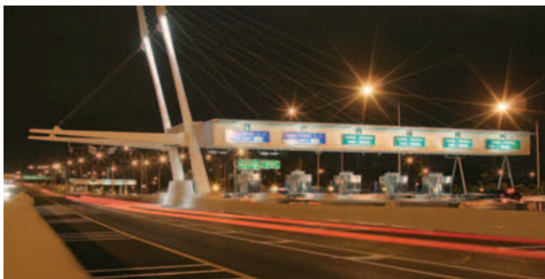
ORT uses overhead gantries like the one on SR 836 which enables drivers to pay tolls while maintaining highway speed.
